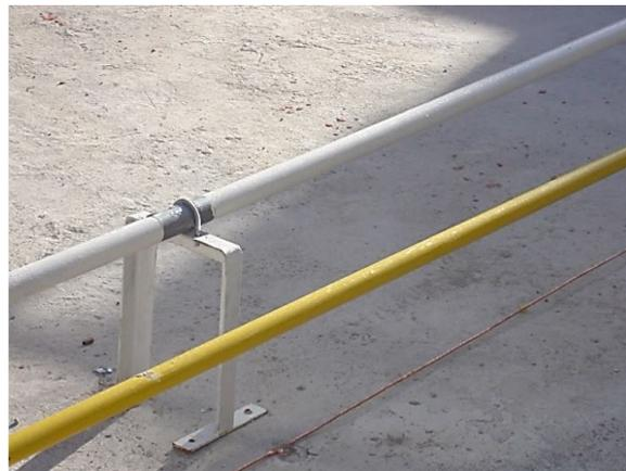
Figure 5. Signaling of LPG pipes (yellow LPG vapor, white LPG liquid).
