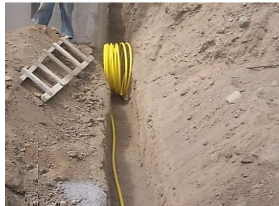
Figure 2. Polyethylene pipe ready to be installed.
